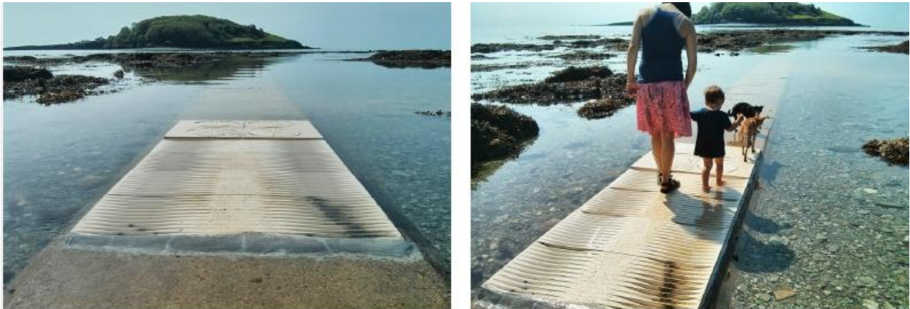
Figure 10 Eco-enhanced stormwater outfall at Hannafore beach
