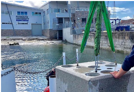
Figure 6 BIOBLOCK being lifted into place [Source: https://www.plymouth.ac.uk/news/bioblocks-show-how-coastal-designs-could-benefit-marine-life ]
